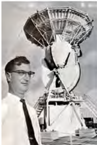
Tracking station director R.P. Jacomb (STADIR is his 'short' title) takes a breather near one of his responsibilities, a 30ft Apollo unified S-Band system scanner which belts out up to 20kw of power.
