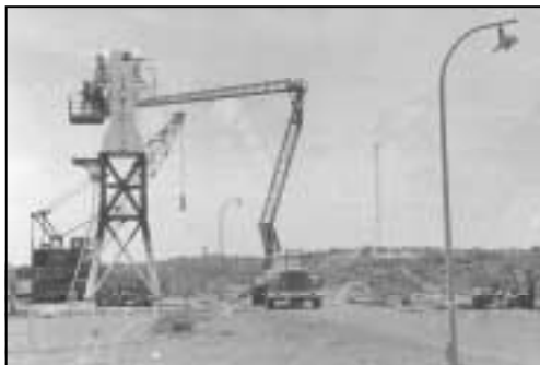
Removing Range and Range Rate Antenna
