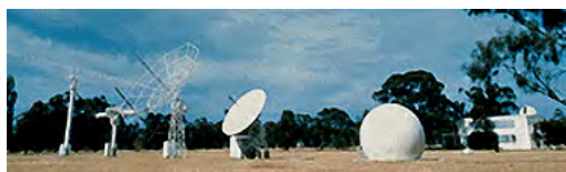
Calgoora Razdow Installation
